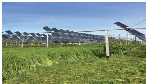
Advanced photovoltaic farm at New Holland Agriculture; panels help to prevent water evaporation
